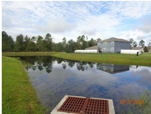
Pond 12: Pond in good condition, no algae noticed.
